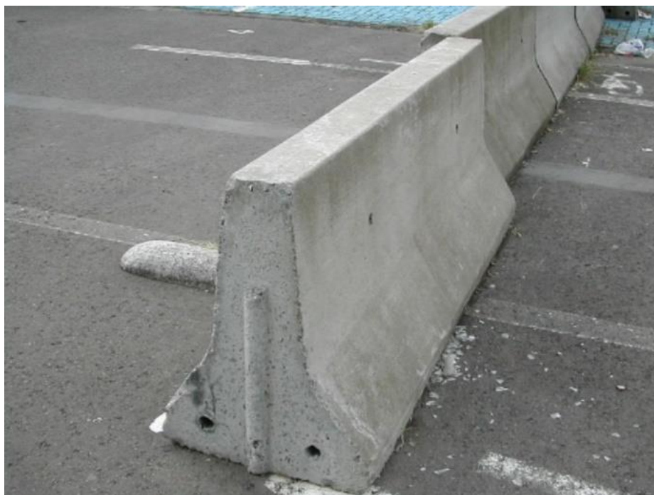
FIGURA 3 – Barreira new jersey
