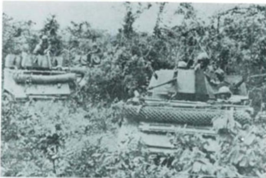
ARMORED CAVALRY ASSAULT VEHICLES WITH RPG SCREENS ON FRONT
