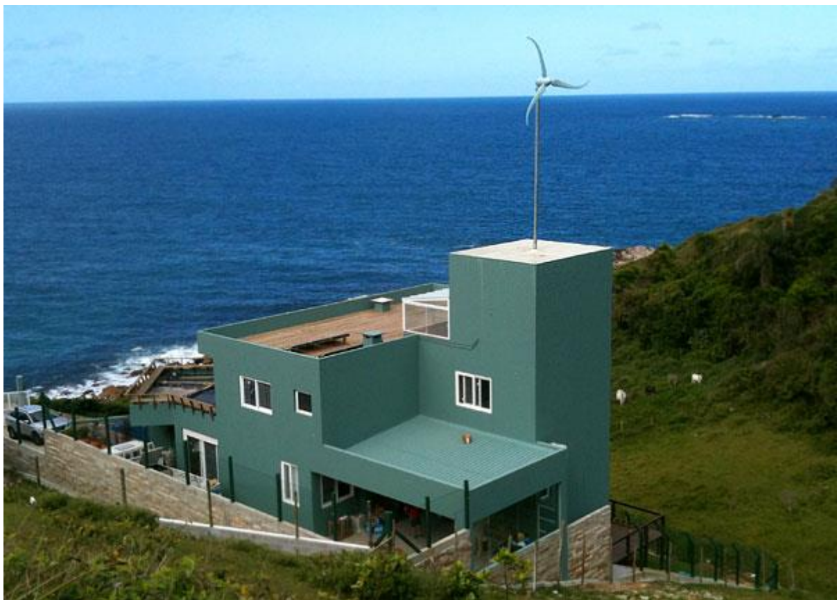
FIG 3.7 – Aerogerador Skystream Land
